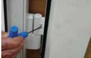
2. To adjust the door horizontally (L to R) open the door & push in the plastic clip
